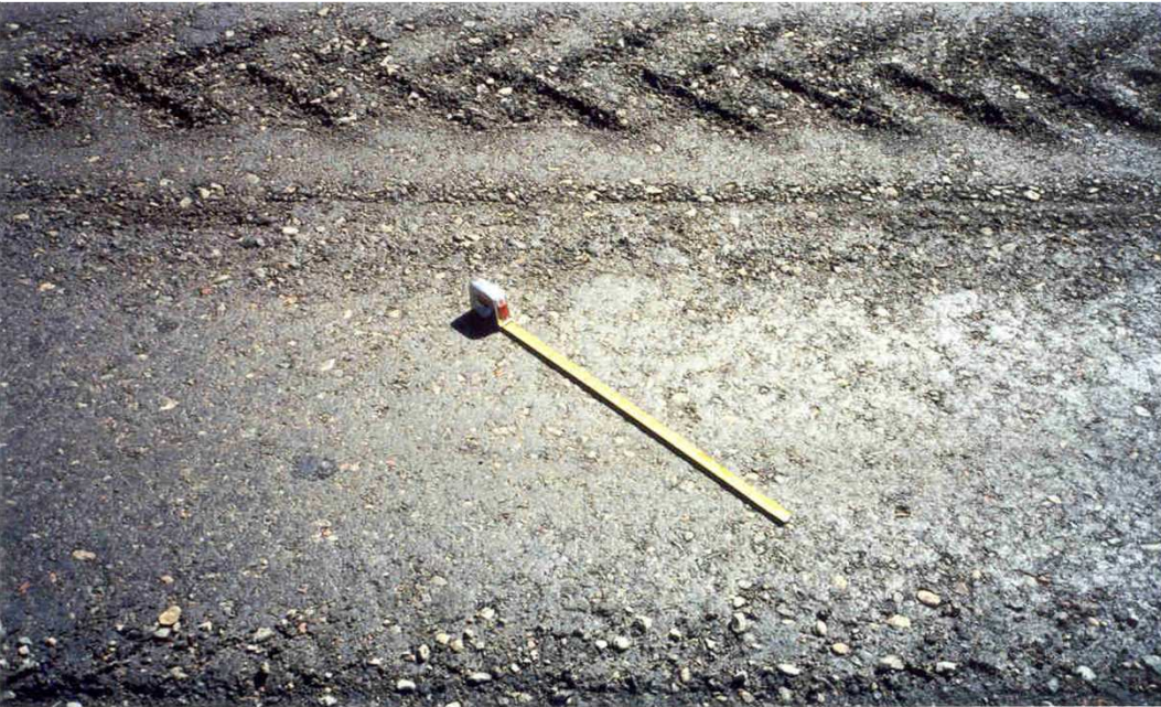
The expanded asphalt mat following initial pass of the breakdown roller
