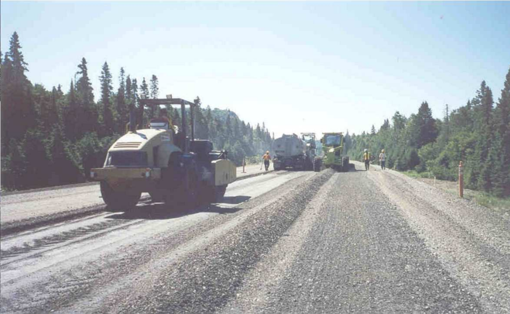
The expanded asphalt mat following initial pass of the breakdown roller
